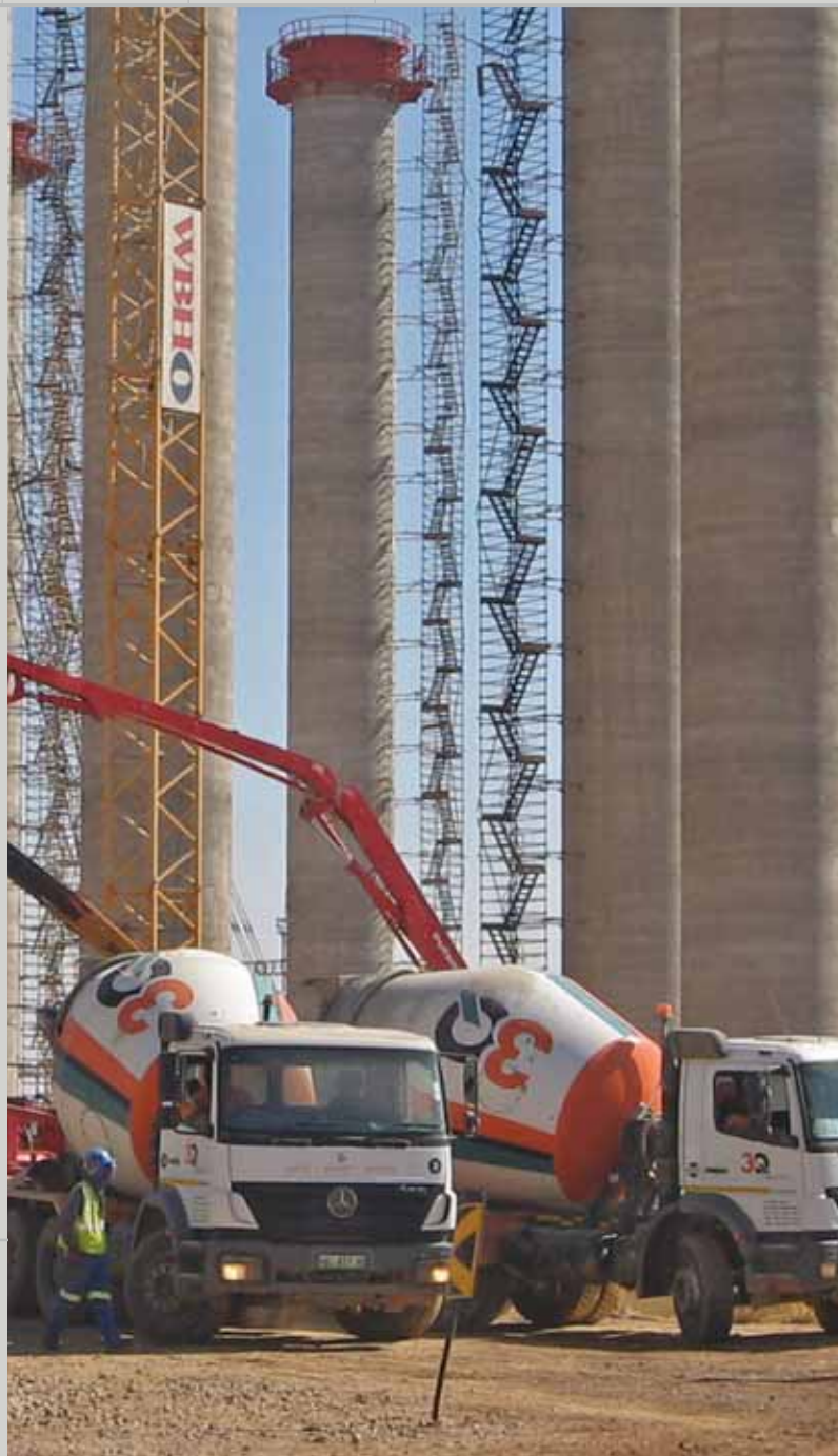
RIGHT 3Q readymix contract at Kusile Power Station
