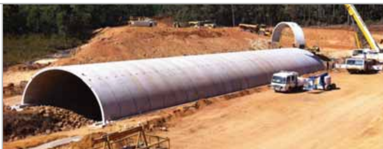
RIGHT Large diameter culvert at Myara WBHO Civil
